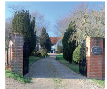
West Bowers Hall, Listed Grade II*
